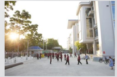
PANDORA production facility in Thailand
